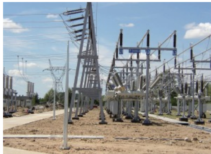
Double busbar arrangement
