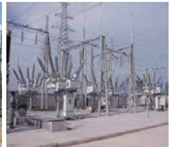
Single busbar arrangement
